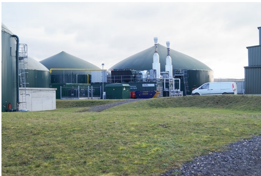
Agrivert's Wallingford anaerobic digestion facility
